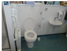
No contrast between walls and fittings, vertical grab bar missing from other side of sink and alarm cord tied
